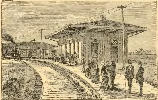
RAILWAY STATION, BOUND BROOK LINE.
